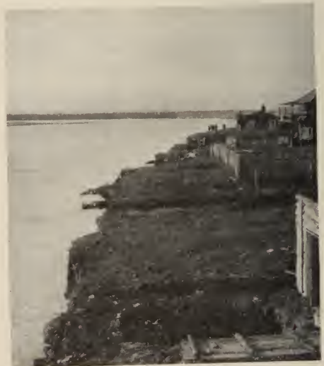
The fence in the right background surrounds our mission property. The projections reaching out over the river are the foundation timbers of a house which has been washed away.
